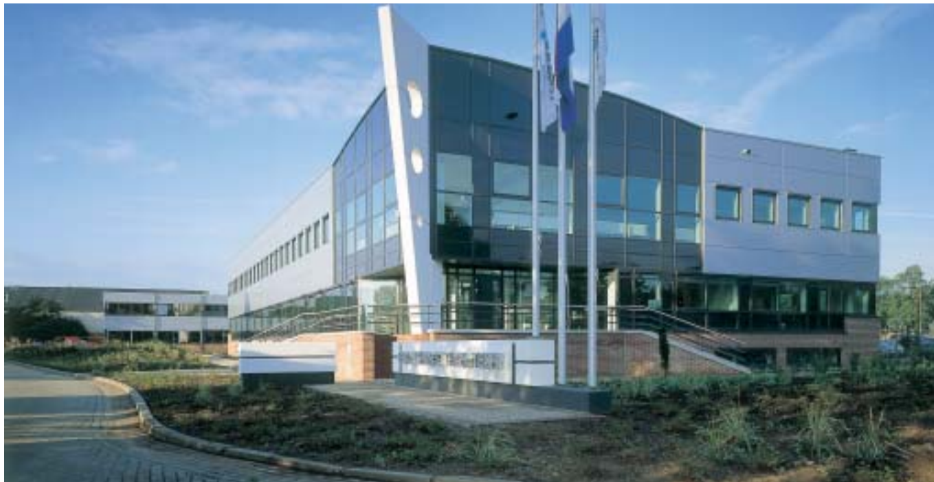
BRONKHORST HIGH-TECH HEADQUARTERS, THE NETHERLANDS
